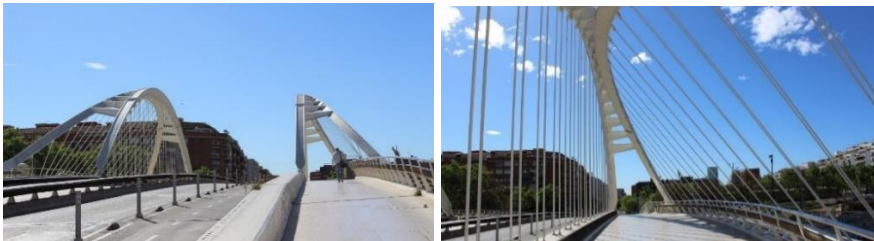
Figure 1.7. Views form Bac De Roda Felipe II Bridge (Kutlu, 2016)
