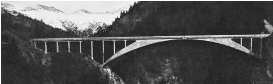
Figure 1.3. Salginatobel bridge view (Billington, 1974; p62)
