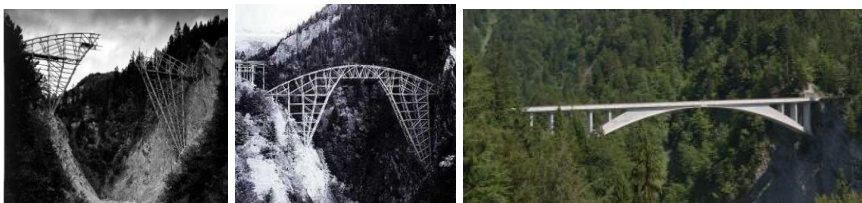
Figure 1.4. Salginatobel bridge construction (Tapping, 2007)
