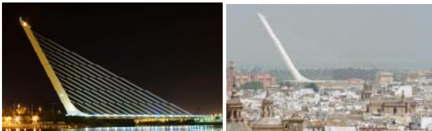
Figure 1.9. Alamillo Bridge views (Orr, 2008; p2)
