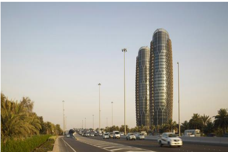
Picture 2.4. Al-Bahr towers in Abu Dhabi (URL 6)
