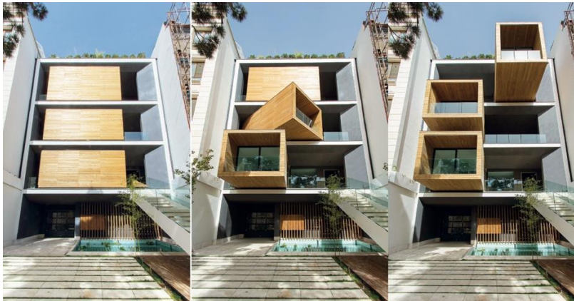
Picture 2.9. Sharifi-Ha House facade (Sojoudihassanlouei, 2019).
